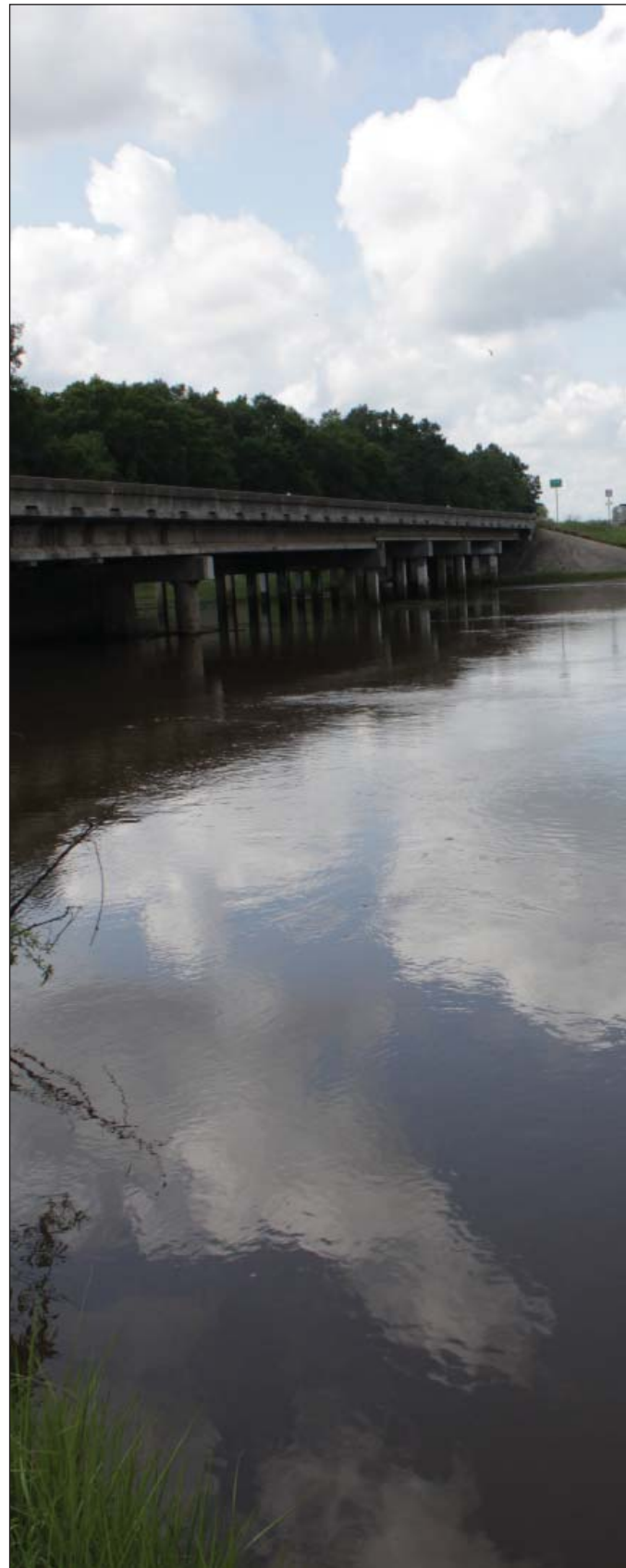
Flooding on the Neches River at US 59 in Diboll, June 10, 2016
