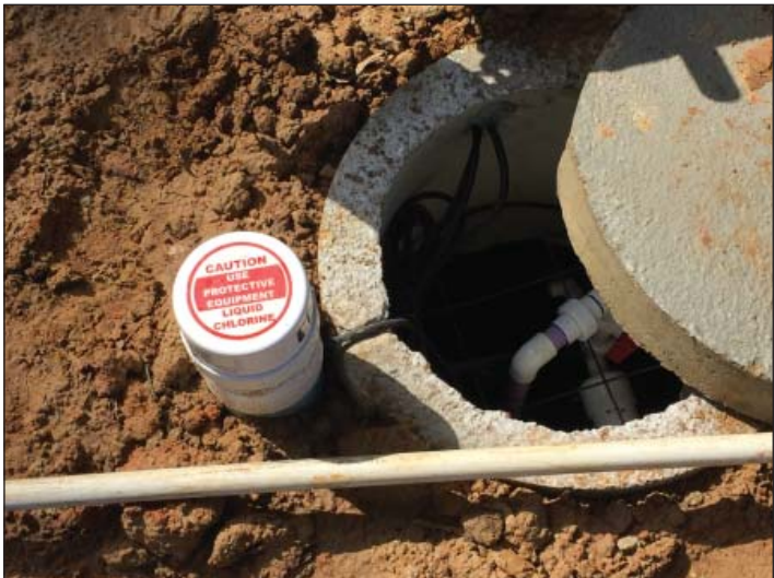
Aerobic OSSF systems installed in the Attoyac Bayou Watershed
