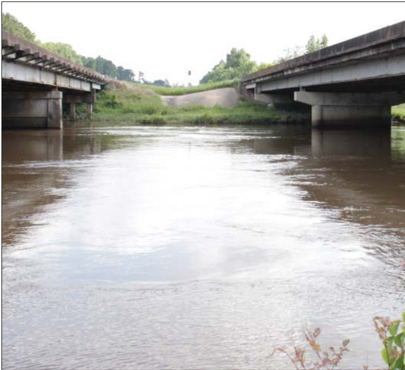
Flooding on the Neches River at US 59 in Diboll, June 10, 2016
